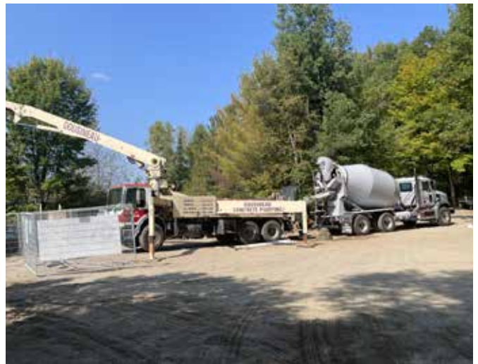
Concrete work at the dam. Photo by MNRF
